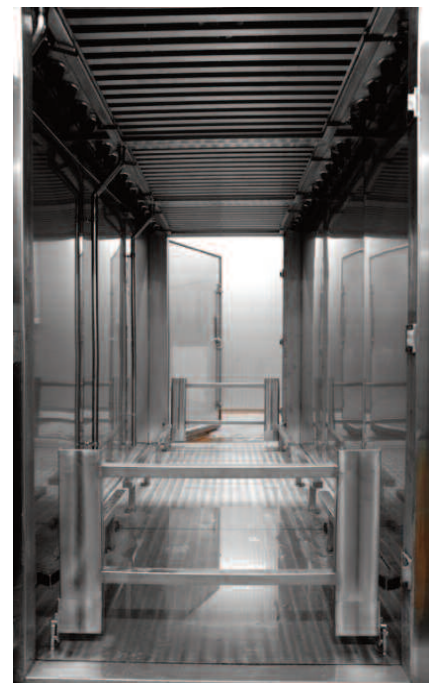
Inside Smokehouse with Ramps Up
